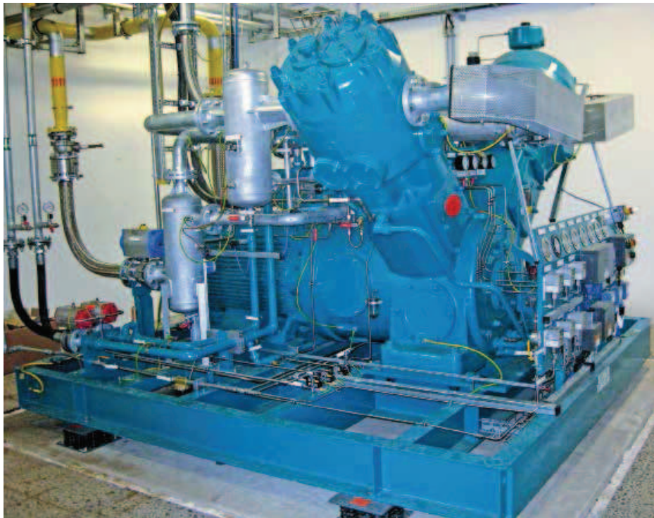
Fig. 2: Compressor plant for biomethane grid injection
